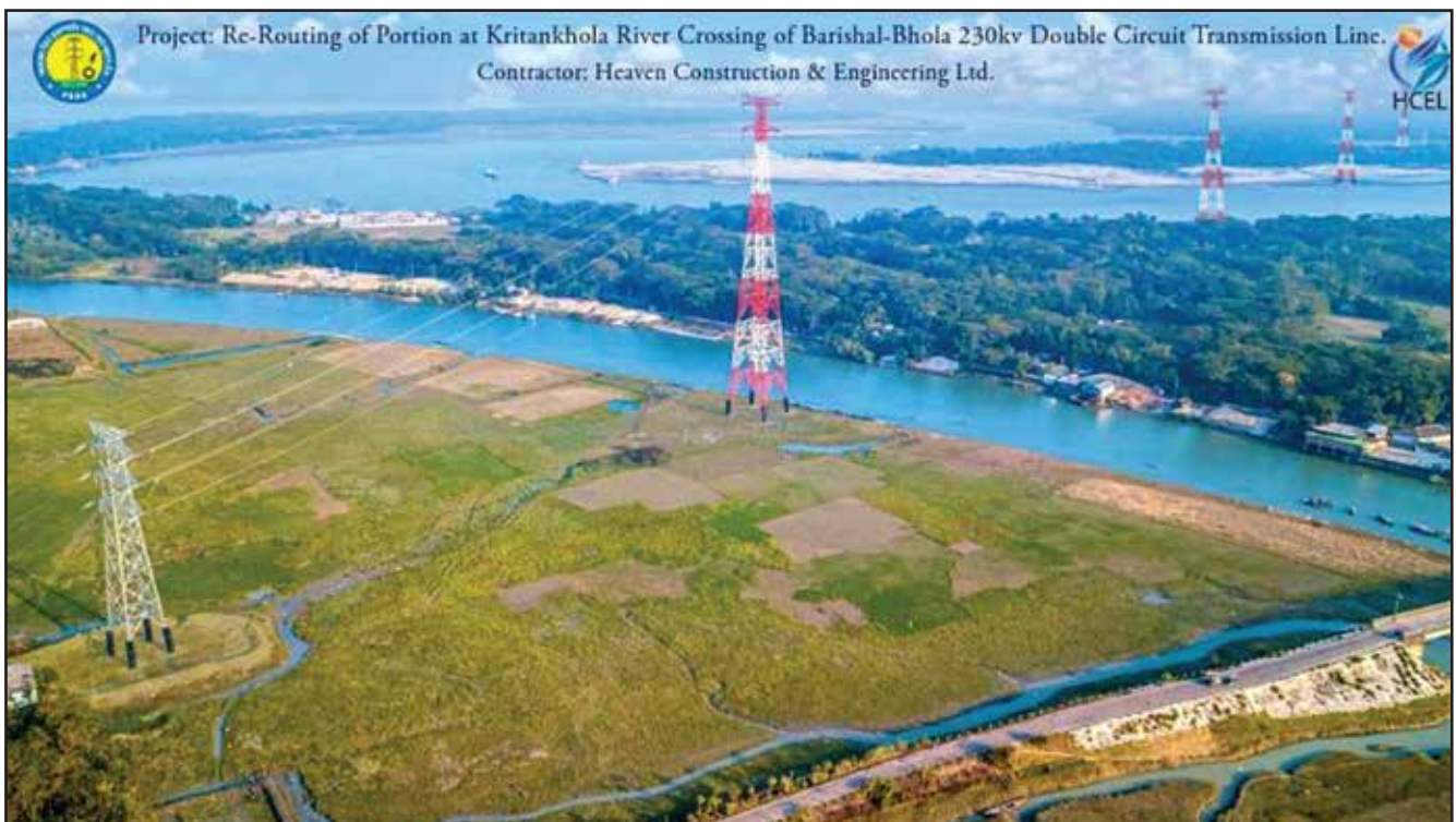
MMBPLC Financing infrastructure
